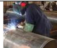
**SOLDADURA DE TUBERÍA CON PROCESOS SEMIAUTOMÁTICOS GMAW-S (RMD™), GMAW-P (PRO-PULSE™) Y FCAW-G**
